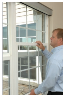
2. Lift sash above clips
