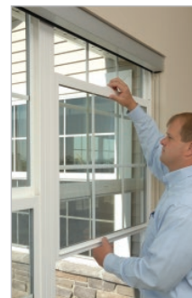
3. Shift sash to right within channel
