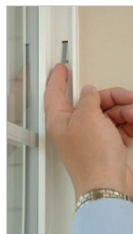
7. Insert sash into channel above clips
