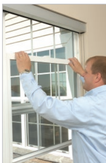
8. Lower sash to sill
