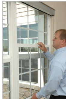
2. Lift sash above clips
