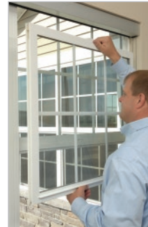
7. Insert sash into channel above clips
