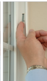
7. Insert sash into channel above clips
