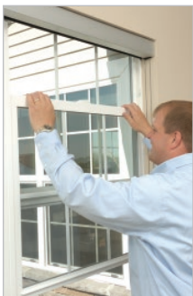
8. Lower sash to sill
