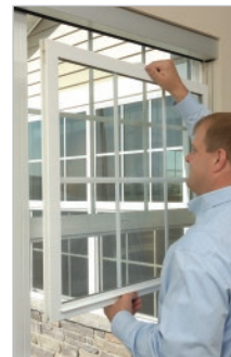
7. Insert sash into channel above clips
