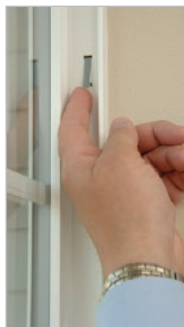
7. Insert sash into channel above clips
