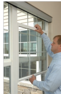
3. Shift sash to right within channel
