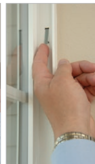
7. Insert sash into channel above clips
