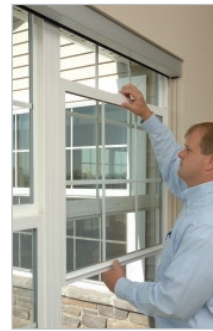
3. Shift sash to right within channel
