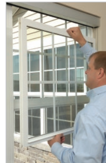
7. Insert sash into channel above clips
