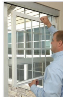
7. Insert sash into channel above clips
