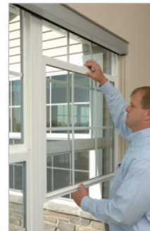
3. Shift sash to right within channel
