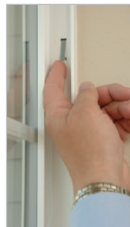
7. Insert sash into channel above clips
