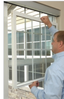
7. Insert sash into channel above clips
