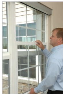
2. Lift sash above clips
