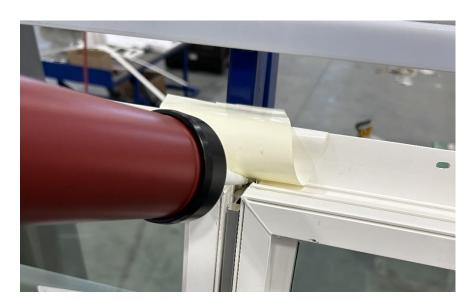
9) Apply a 1/8" bead of silicone to each unit in the exterior frame accessory groove as shown below:
