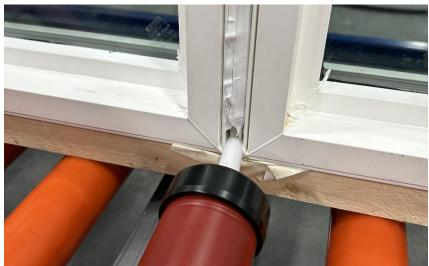
14) Apply a 1/8" bead of silicone to interior frame accessory groove.
