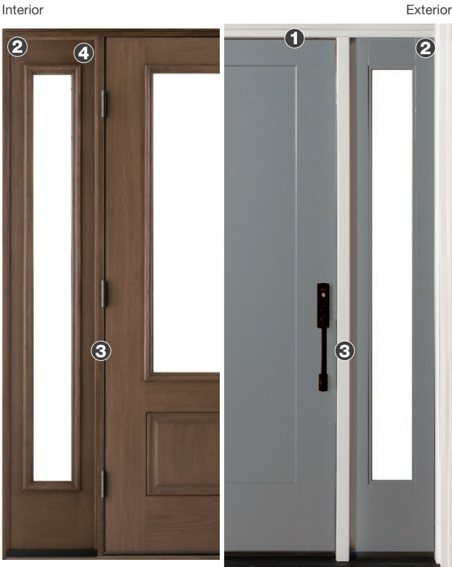
1 Brickmould 2 Jamb 3 Mullions 4 Cove Mould
